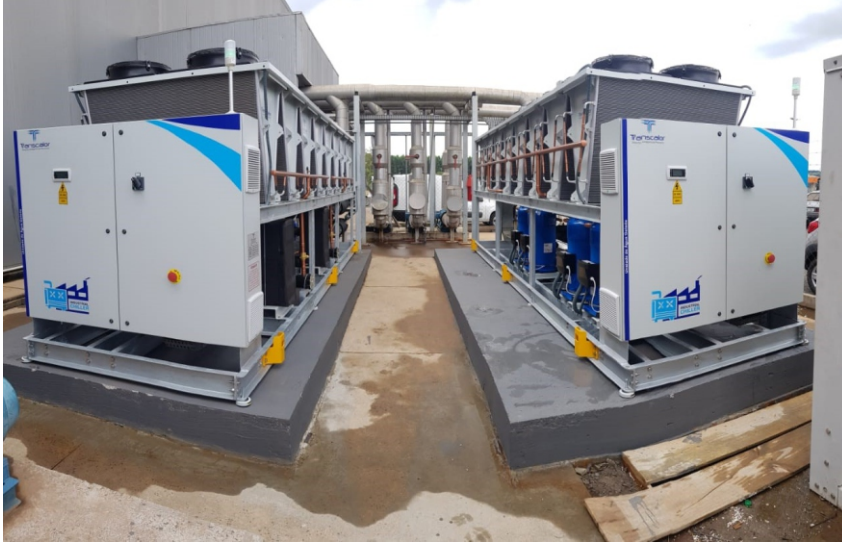
Transcalor's TRA 480 Chiller with SWEP P250AS models installed.
